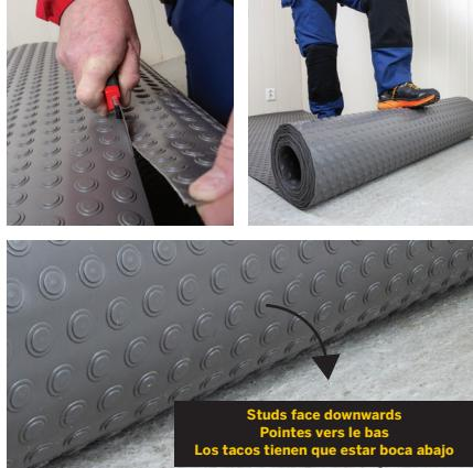
**1.** Measure, cut, and dry fit the first section of M-D MULTI-FLOOR®, ensuring the studs are facing down.
