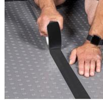
**3.** Seal all joints with M-D MULTI-FLOOR® SEALING TAPE.
